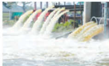
Polluted sewerage water Water pollution
